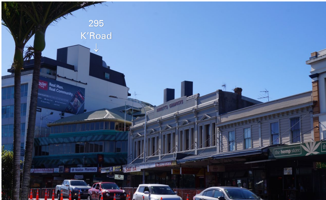
Figure 6 - Karangahape Road streetscape showing buildings near to the Site
